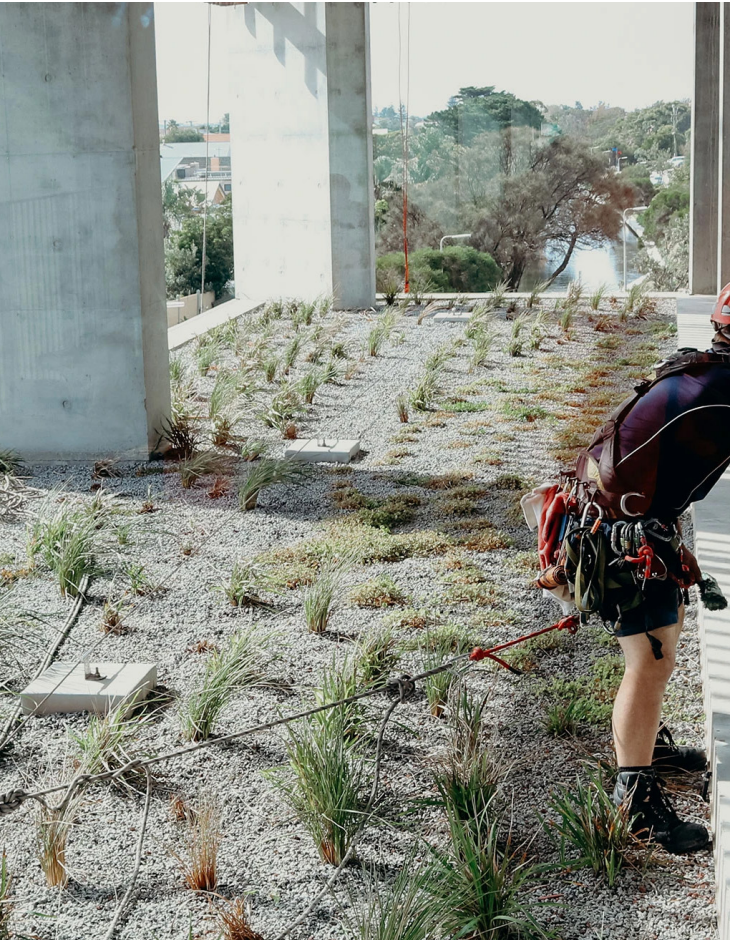
Example of static line fall arrest system
